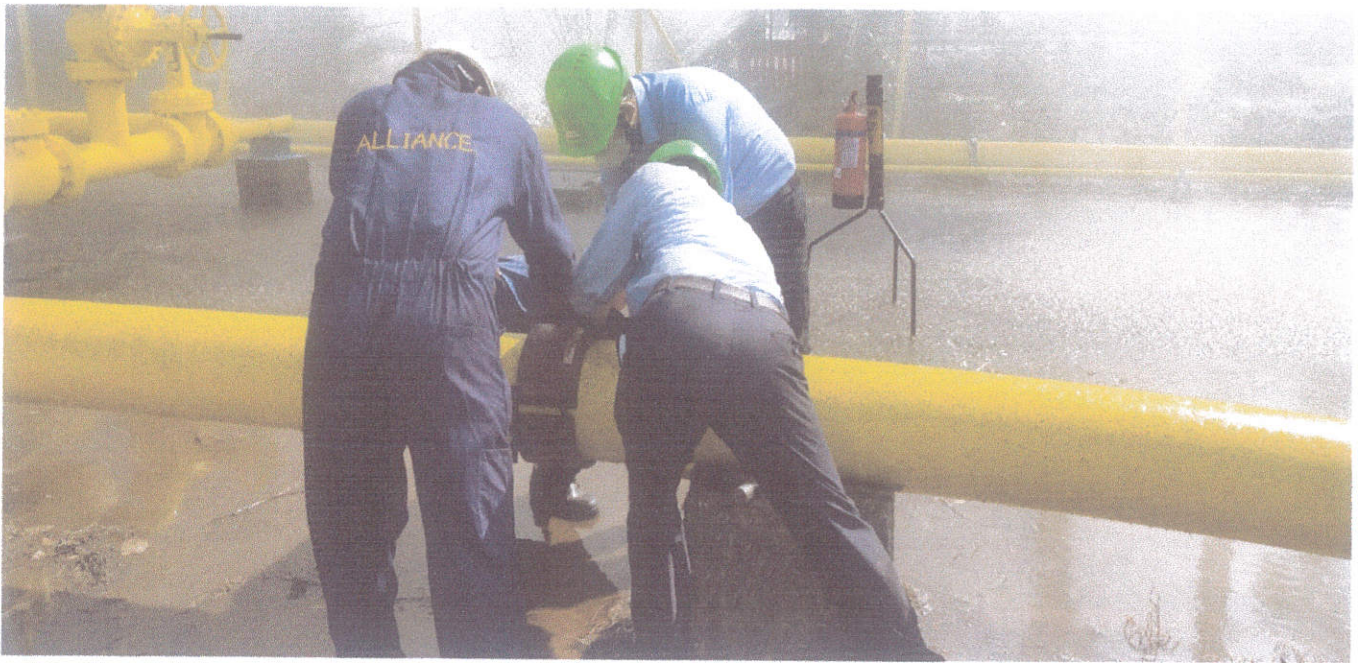
Mayura curtain/Water Spray started to Disperse/Contain the gas
