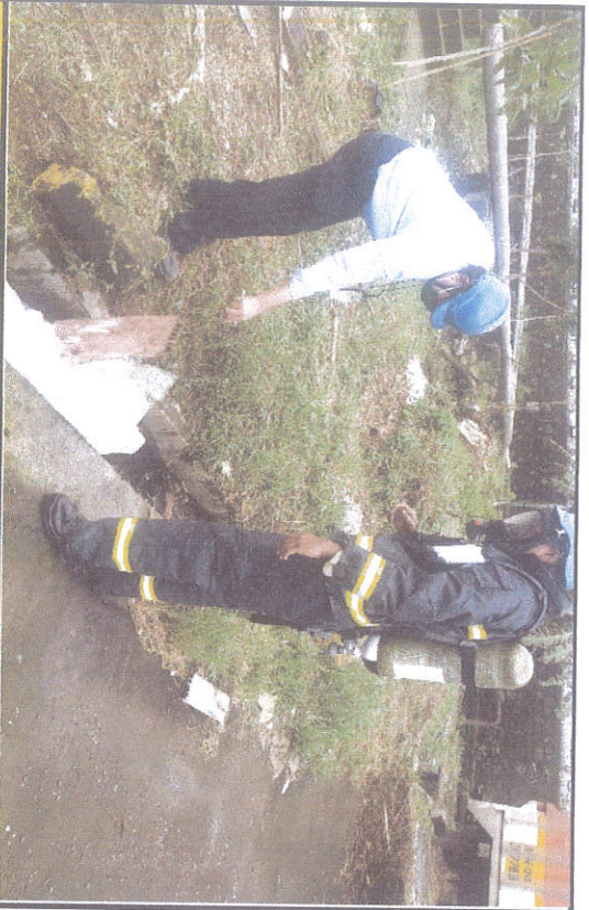
Bundling arrangement done on storm drain to contain the IPA spillage
