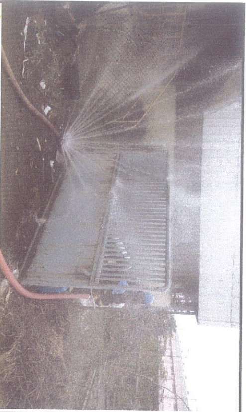
Water Mayura curtain operated to contain the radiation Heat
