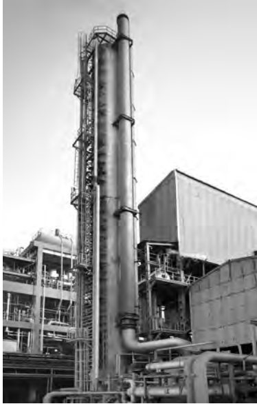
Nitric Acid plant, Taloja
