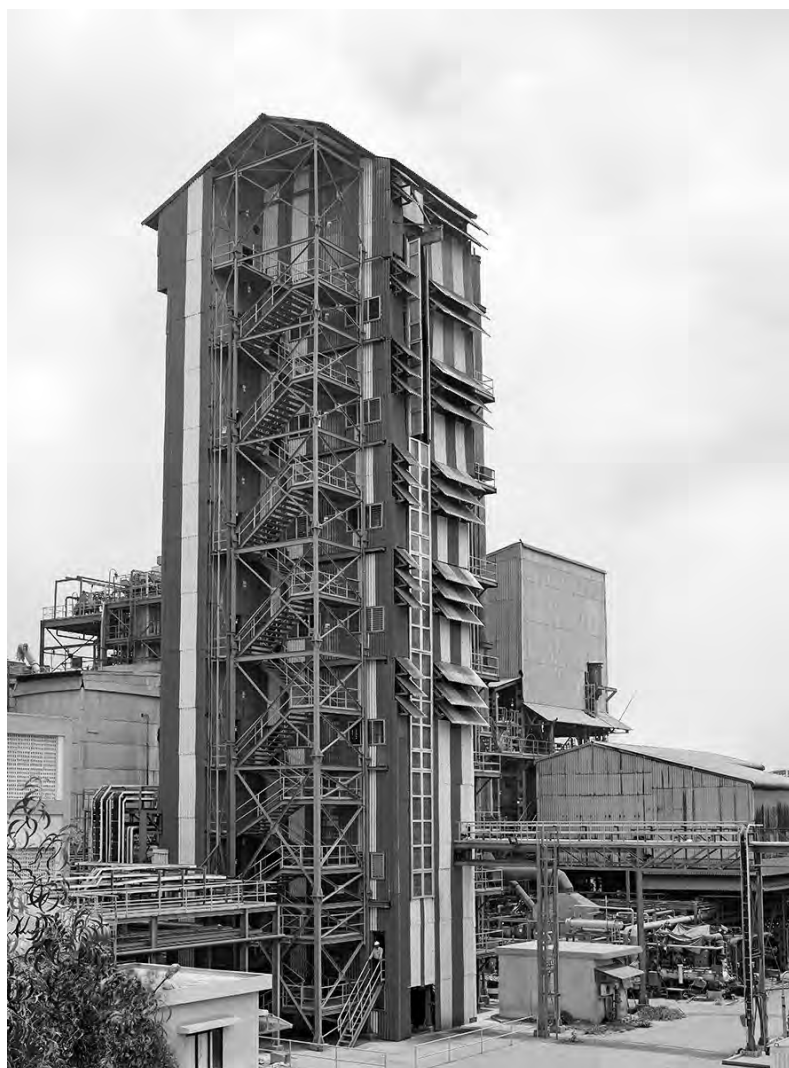
Nitric Acid plant, Dahej
