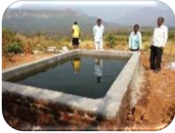
Support for water resource development and conveyance
