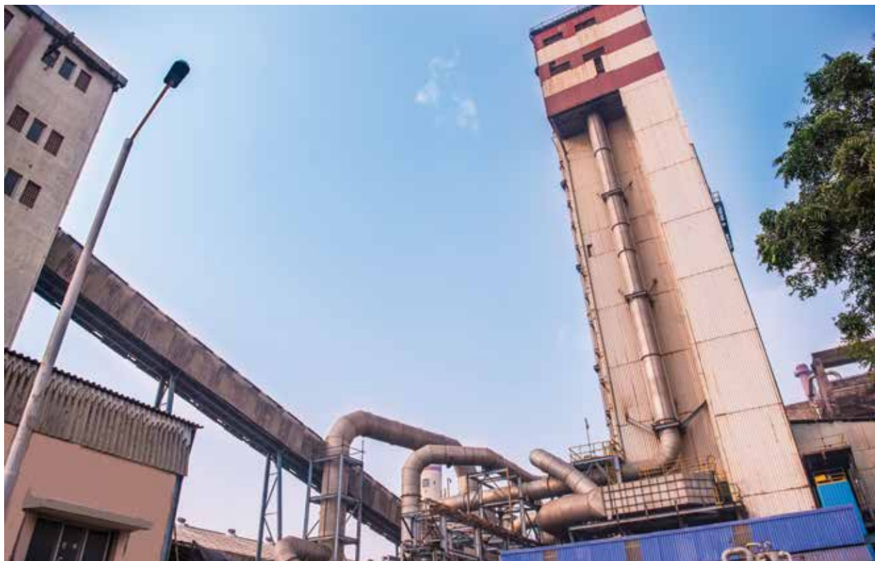
Prilling Tower at Taloja
