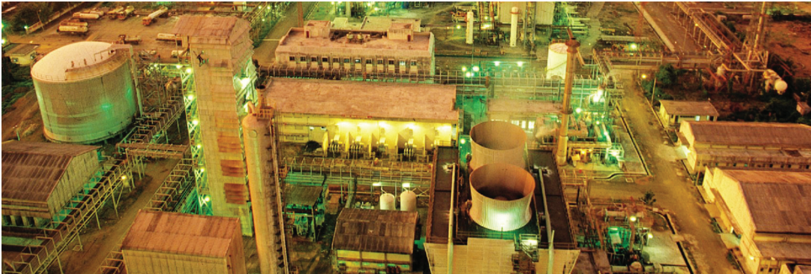
A BIRD'S EYE VIEW OF DFPCL'S PLANT AT TALOJA NEAR MUMBAI.
